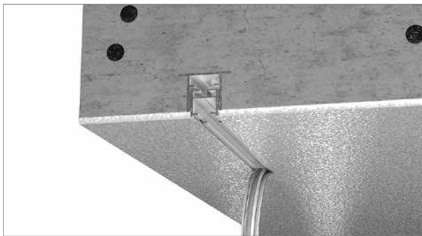
13. Remove the strip when the plaster is still wet.
